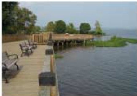
Bridges over creeks that flow into the river
