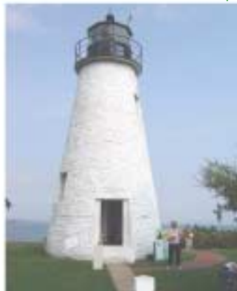
Historic Structures along the riverfront
