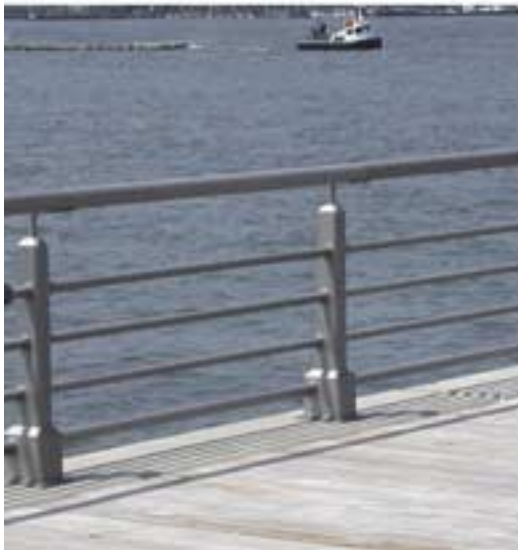
Guardrail at river's edge
