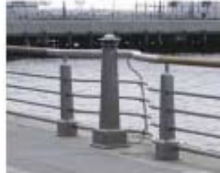
Guardrail with integral lighting
