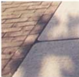
Brick with Stone Pavers
