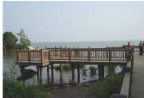
Wood-frame observation pier
