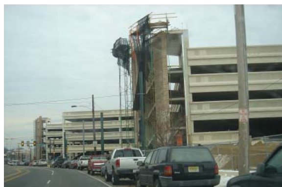
Construction of new parking garage by SEPTA Bustleton Ave. near FTC
