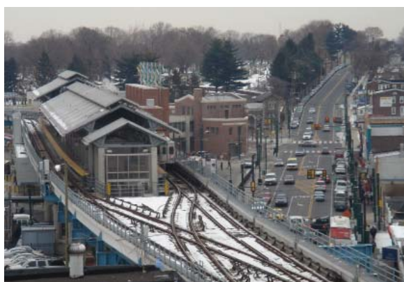
Realigned El structure and Frankford Avenue
