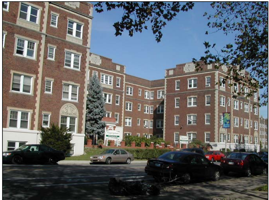
The newly renovated Chatham Court Apartments at SW corner 49 th & Locust: publicly-assisted and developed by The Partnership CDC.
